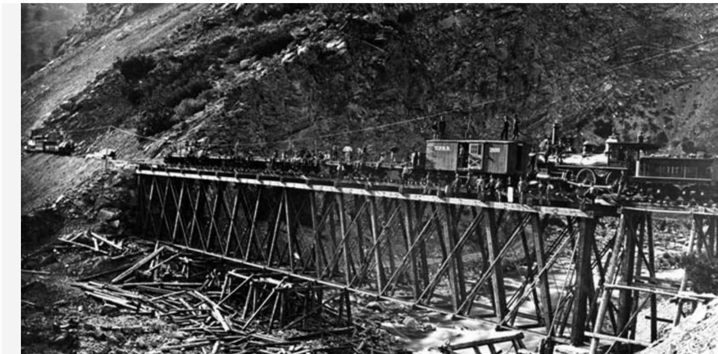
Image 12.3 Photo of Union Pacific Railroad Bridge Under Construction
