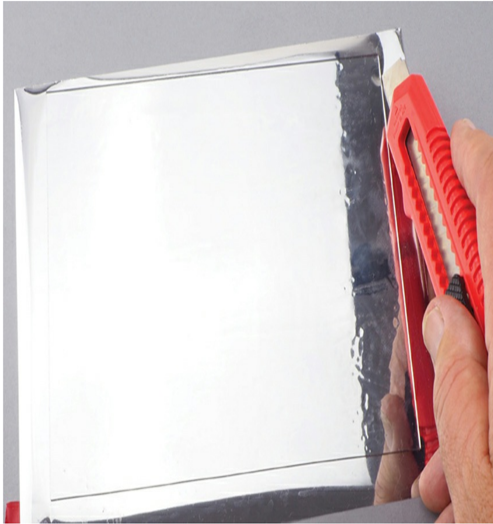
Figure 3-16: Trimming the reflective window film
