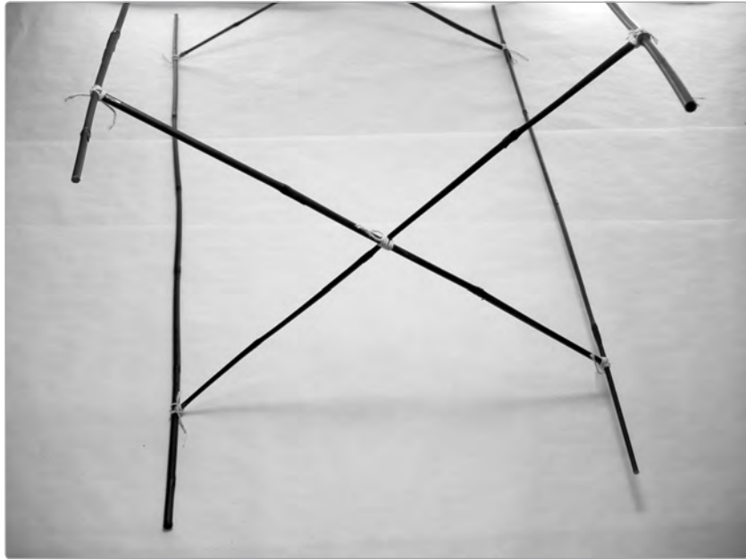
FIGURE 23-19: The top cross braces secured with string
