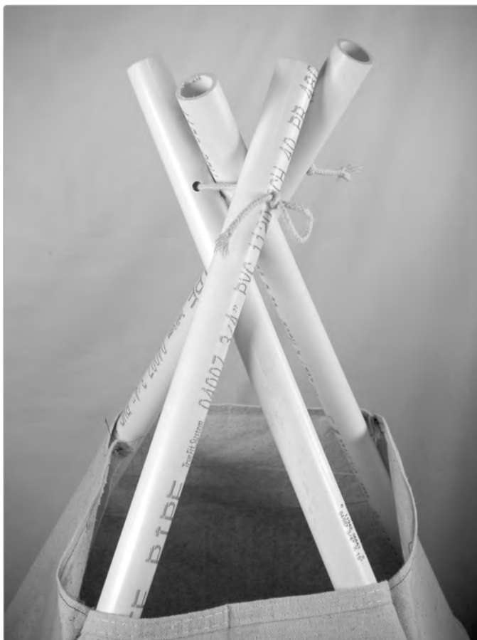
FIGURE 4-15: Detail of the tops of the poles once the teepee is pitched; notice that the cord joining the poles allows for a good deal of play
