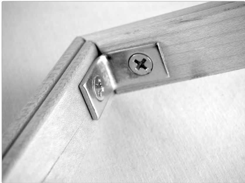
FIGURE 9-5: Detail of an inner frame corner brace
