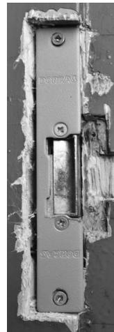
**FIGURE 6-2: THE ELECTROMECHANICAL DOOR LATCH**
