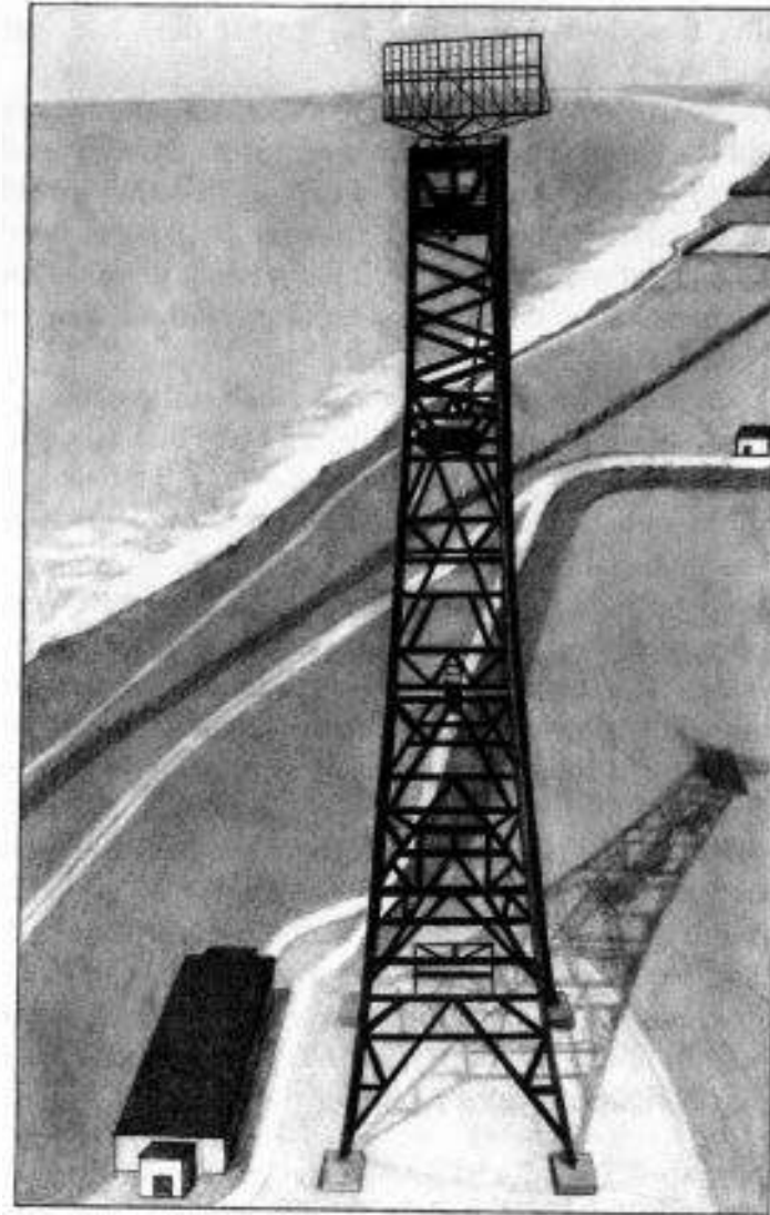
World War II coastal radar station
